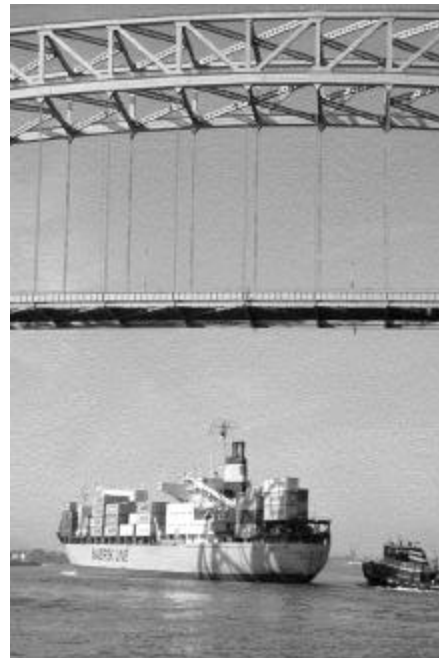
Figure 3 A container ship navigating the Kill Van Kull passing under the Bayonne Bridge. (USACE photo)
