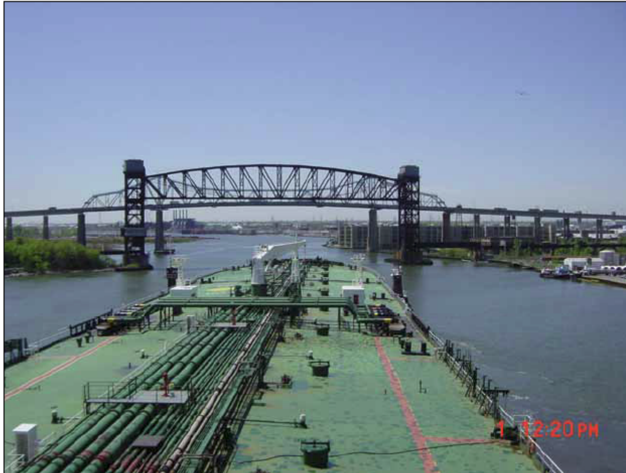
Figure 5. Tromso Trust approaching Bayway Bridge
