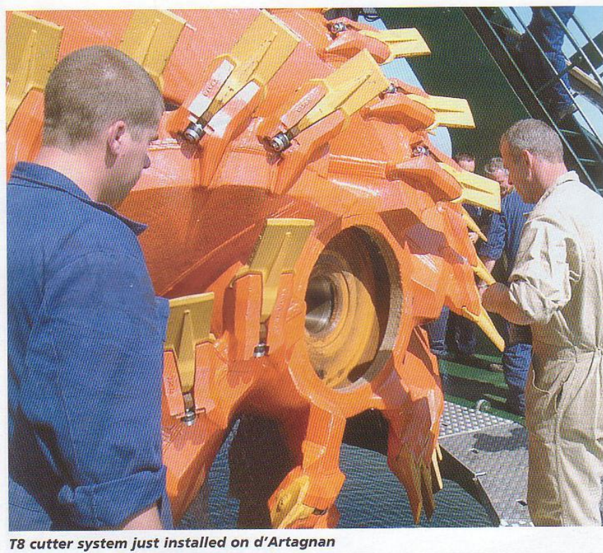
T8 cutter system just installed on d'Artagnan
