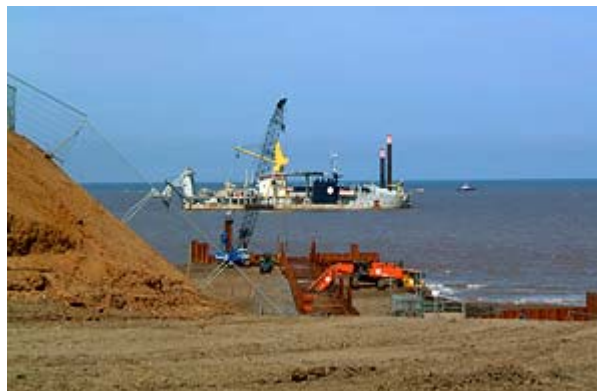
LANGELED LANDFALL: The dredging vessel "JFJ de Nul" started its trenching work - to a point some 20 km off the coast of Easington, England - last week.
