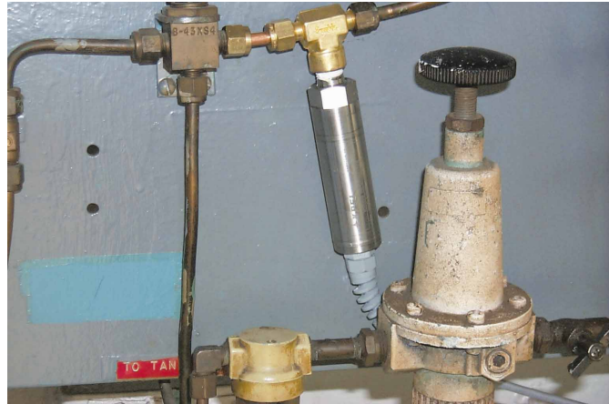
Figure 6. Draft transducer installed in the bubbler line
