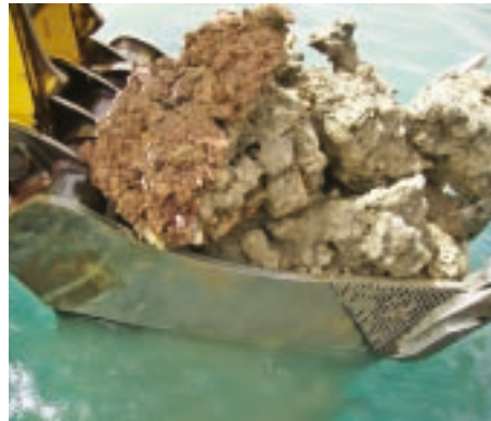
Figure 2. Coral blocks with size up to 2 m excavated by the backhoe dredger.
