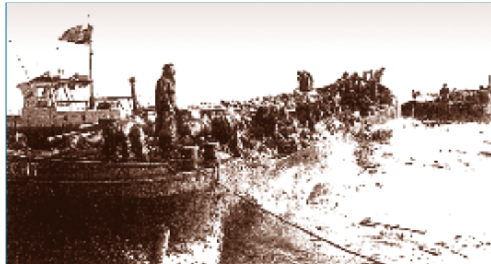
Figure 4. Installation of rock was done from ashore and from a vessel by hand.
