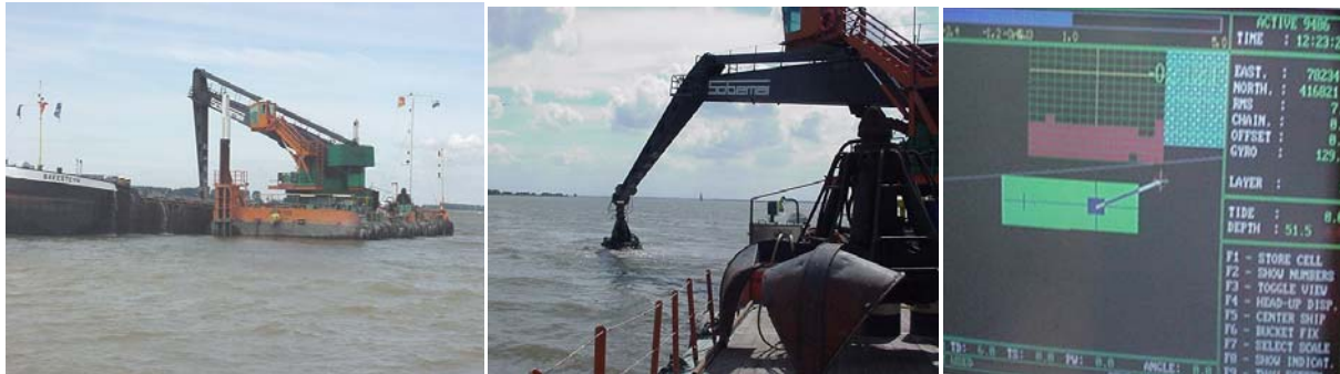
Figure 7: Capping with the grab dredger.
